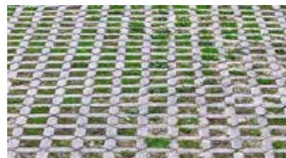
*Concrete and plastic permeable paving*
