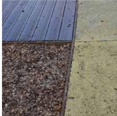
*Boundary between wood chips, decking and pervious concrete using a wooden rail.*
